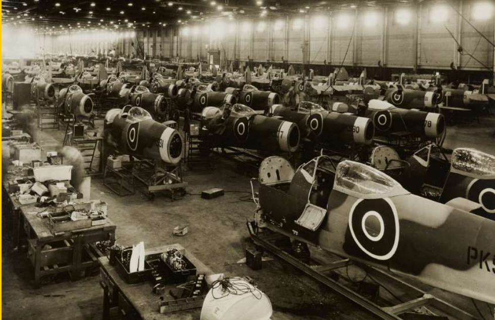
SPITFIRE FINAL ERECTION — FUSELAGE ASSEMBLY (INTERMEDIATE)
